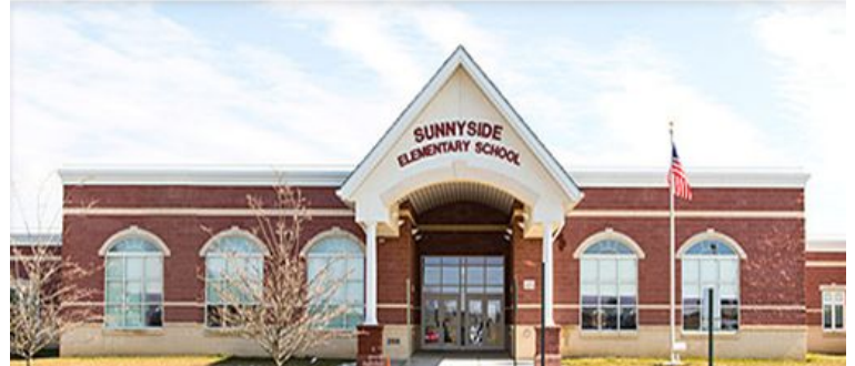
Sunnyside Elementary School
