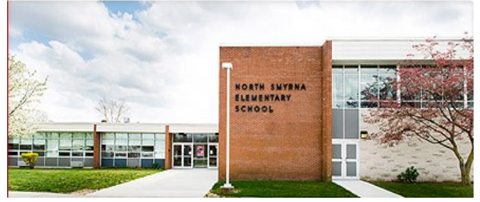
North Smyrna Elementary School
