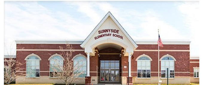
Sunnyside Elementary School
