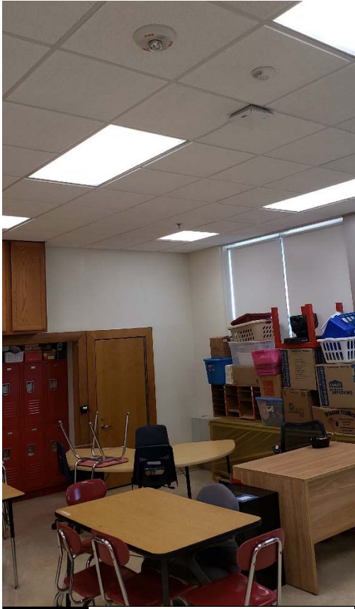
Typical Classroom with 2'x4' Lights and Occupancy Sensor
