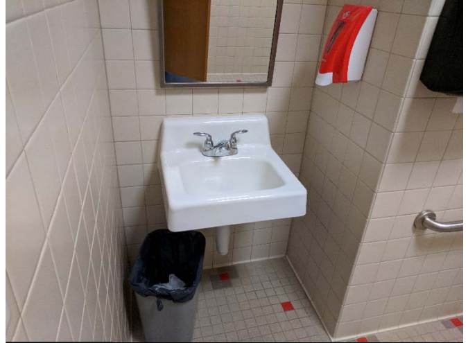
Photo #12 Typical Bathroom Sink
