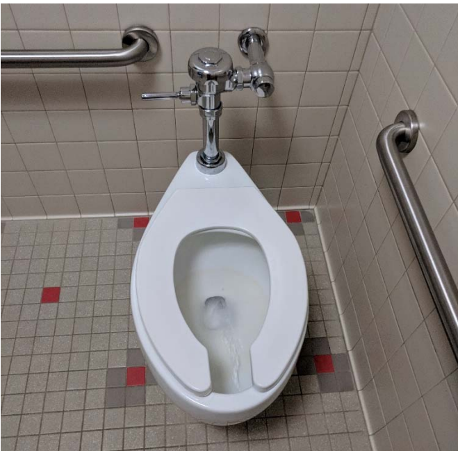
Photo #13 Typical Bathroom Toilet
