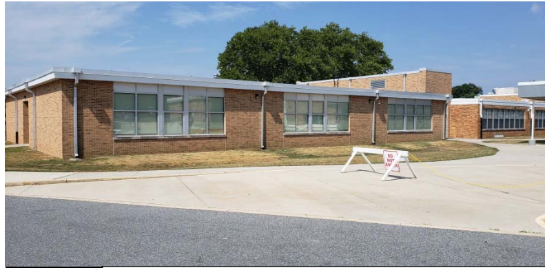
Photo #1 Exterior of 2006 Addition
