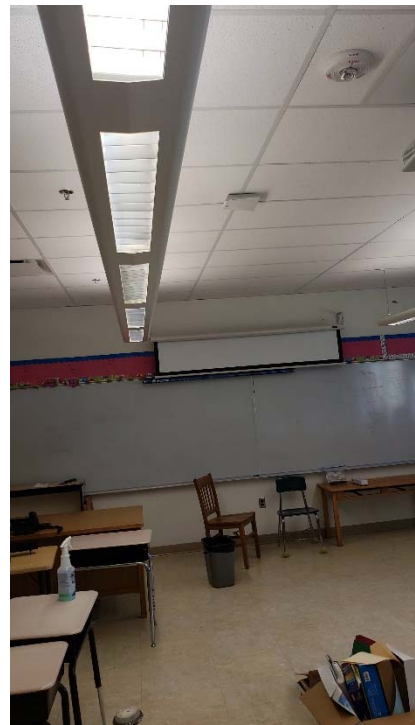
Photo #9 Typical 2006 Addition Classroom
