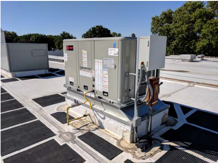
AHU-2 Rusted Disconnect Switch
