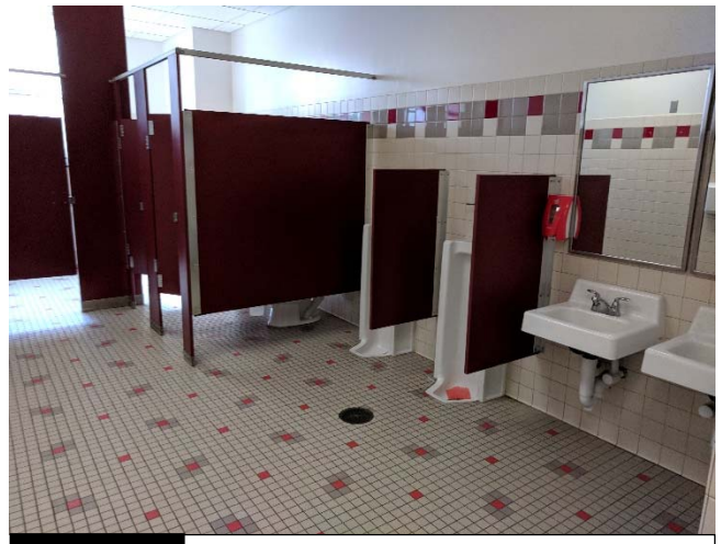
Photo #14 Typical Bathroom
