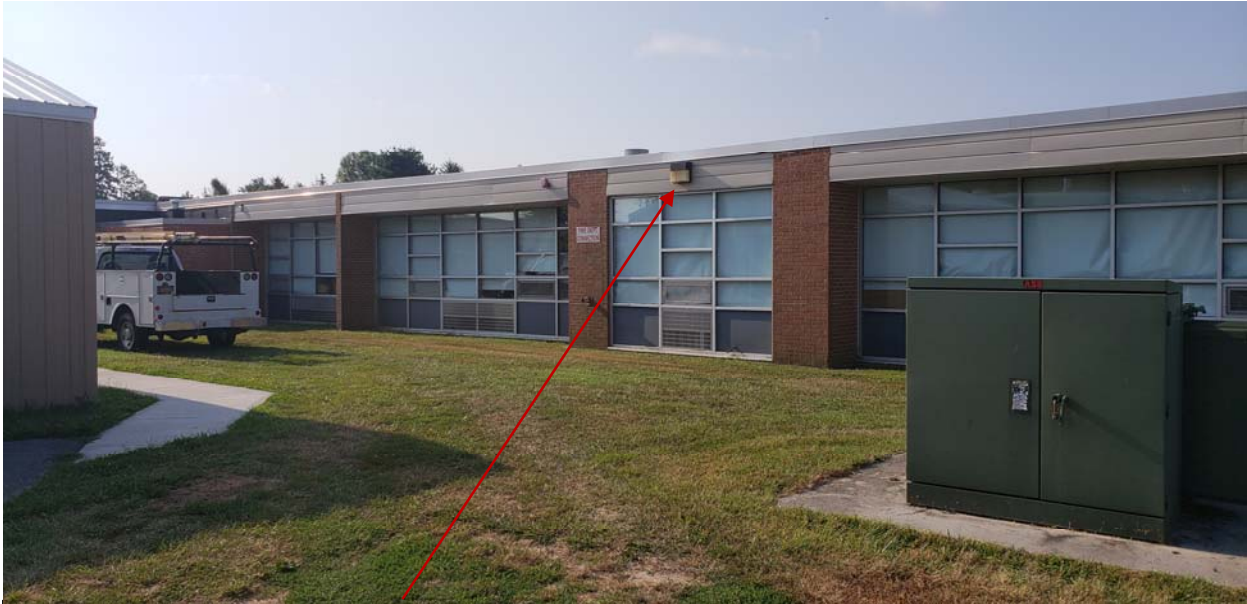
Photo #22 Typical Wall pack
