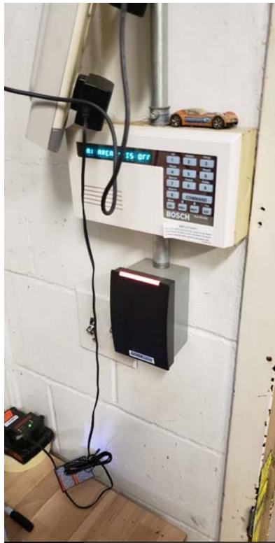
Photo #7 Security Keypad and Card Reader
