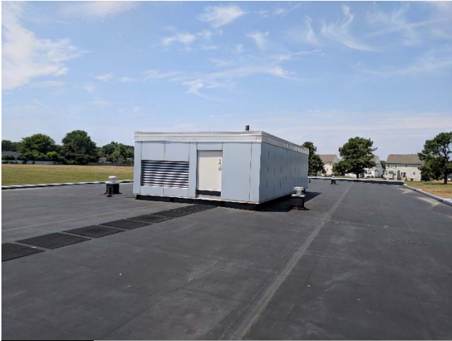
Photo #7 Mechanical Penthouse on Roof
